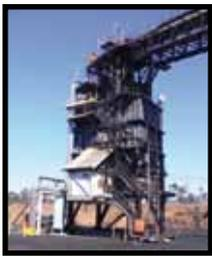
This project is at Goonyella Riverside Mine in the Bowen Basin, where INETE was engaged to manage commissioning of mechanical and electrical components of the mine's enhanced train loadout facility. The project was carried out in five stages over a two-year period, with major works in 2007-08, increasing the loadout capacity from 2500t to 5000t of coal per hour.
