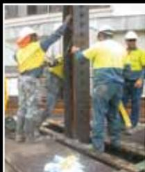
This project demonstrated a superior approach to the design and construction of the foundations for an ocean-front high-rise on the Gold Coast. Research and development on the unique piling requirements for foundations to secure a 77 storey, 277m high apartment tower resulted in reduced bored pile diameters of 1500mm, 1800mm and 2200mm founded up to 45m below the working platform.
