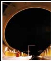
This \$543million project is for design/construction of a seven kilometre dual carriageway highway between Queensland's Gold Coast and northern New South Wales. Work included a 1km tunnel, two major road interchanges, six bridges, and substantial earth works. Significant challenges included building a 'top down' tunnel in a swamp under an airport flight path, adjacent to an environmentally sensitive wetland area and specifically constructing the tunnel 12m below the water table.
