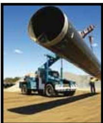
The Alliance investigated, modelled, designed and constructed a series of pipelines that form the South-East Queensland water grid interconnection, a network is capable of transferring up to 217 megalitres of potable water per day. Work covered an area approximately the size of Tasmania and includes 150km of pipelines, six major pump stations, four major reservoirs, four water quality facilities, 21 off-takes and substantial associated infrastructure.
