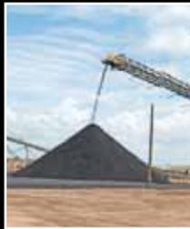
A \$115m project to wash, size and process 5.6 million tonnes of coal a year at Lake Vermont Mine in Central Queensland. Work commenced on site in March 2008 and the project was completed in time by February 2009. Time and resources were saved and safety improved by fabricating large parts off-site, on-ground preassembly of floor sections, and applying Sedgman's innovative Bay Plant design that allowed components to be moved into different design configurations.
