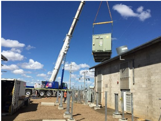
Installation of new drive room:
