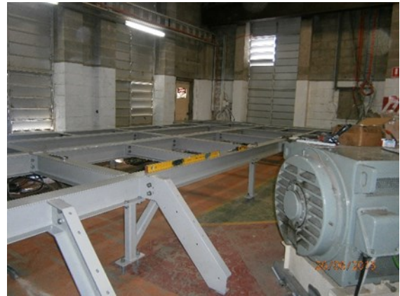
Installation of new switchboard platform:
